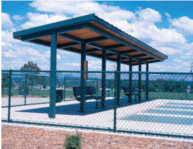
DUG, DUGOUT WITH BURIED FIXED BASE, LITTLETON, CO
